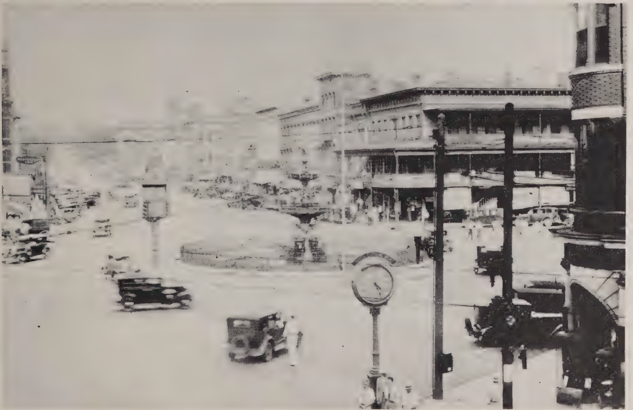
Two views of Court Square looking up Dexter Avenue in 1934. The tower to the left of the fountain was a traffic control tower hand operated during rush hours.
